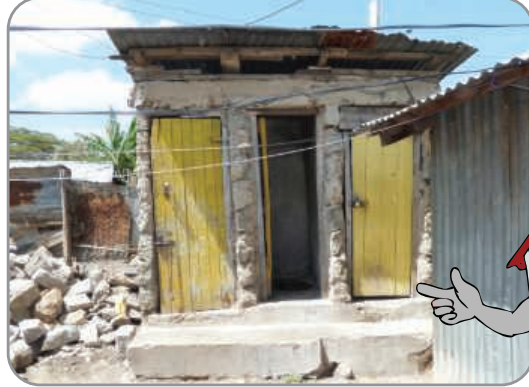
TOILET "B" BEFORE REHABILITATION
