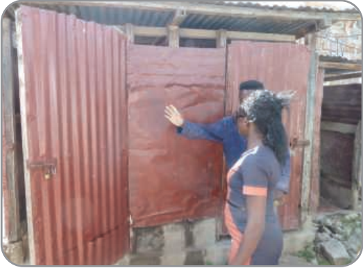
TOILET "A" BEFORE REHABILITATION
