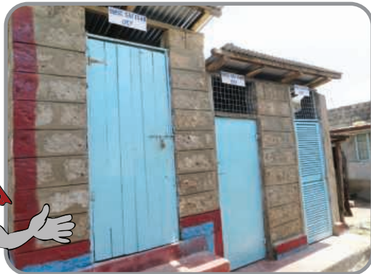
TOILET "A" AFTER REHABILITATION
